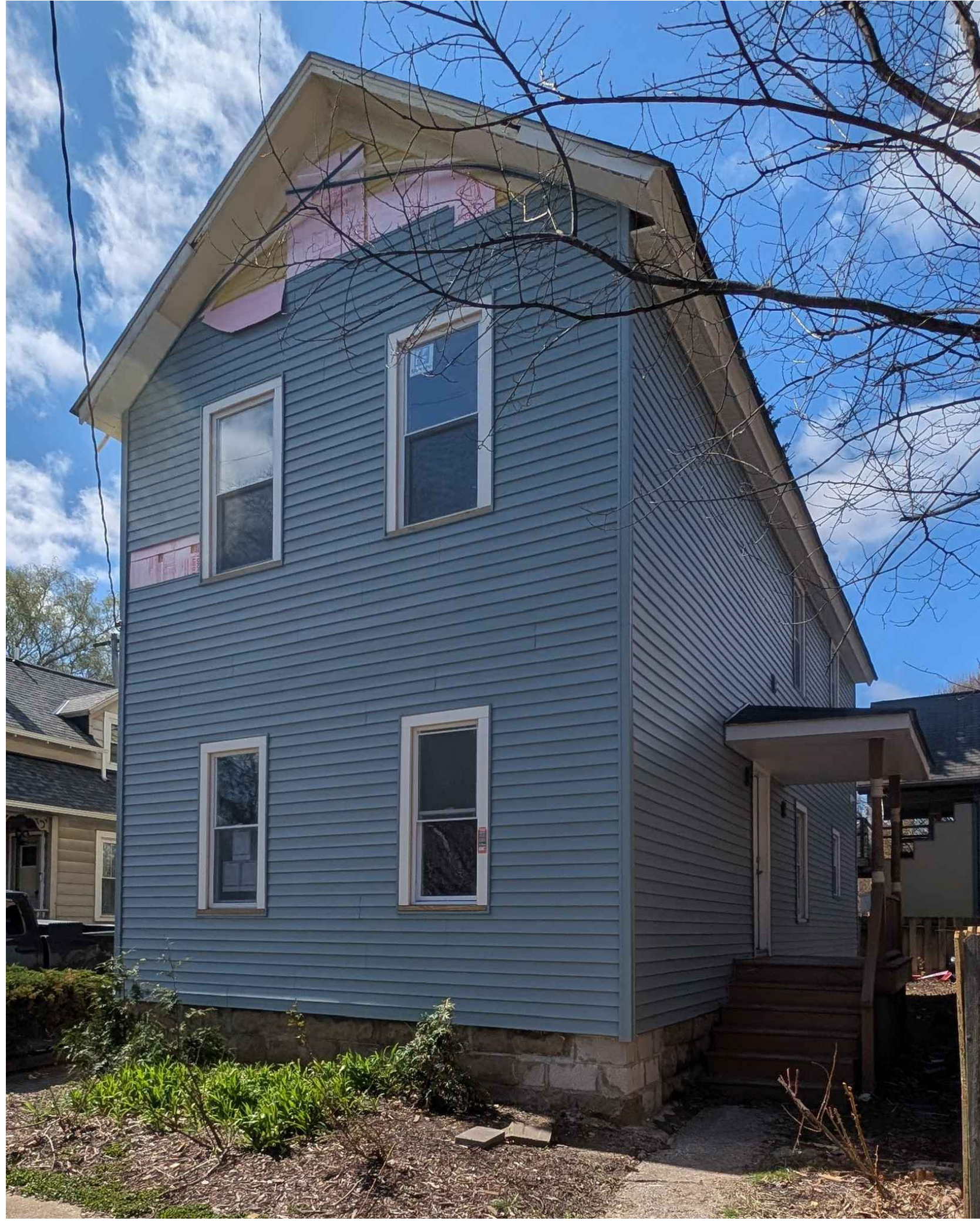
CLOSE UP OF FRONT
