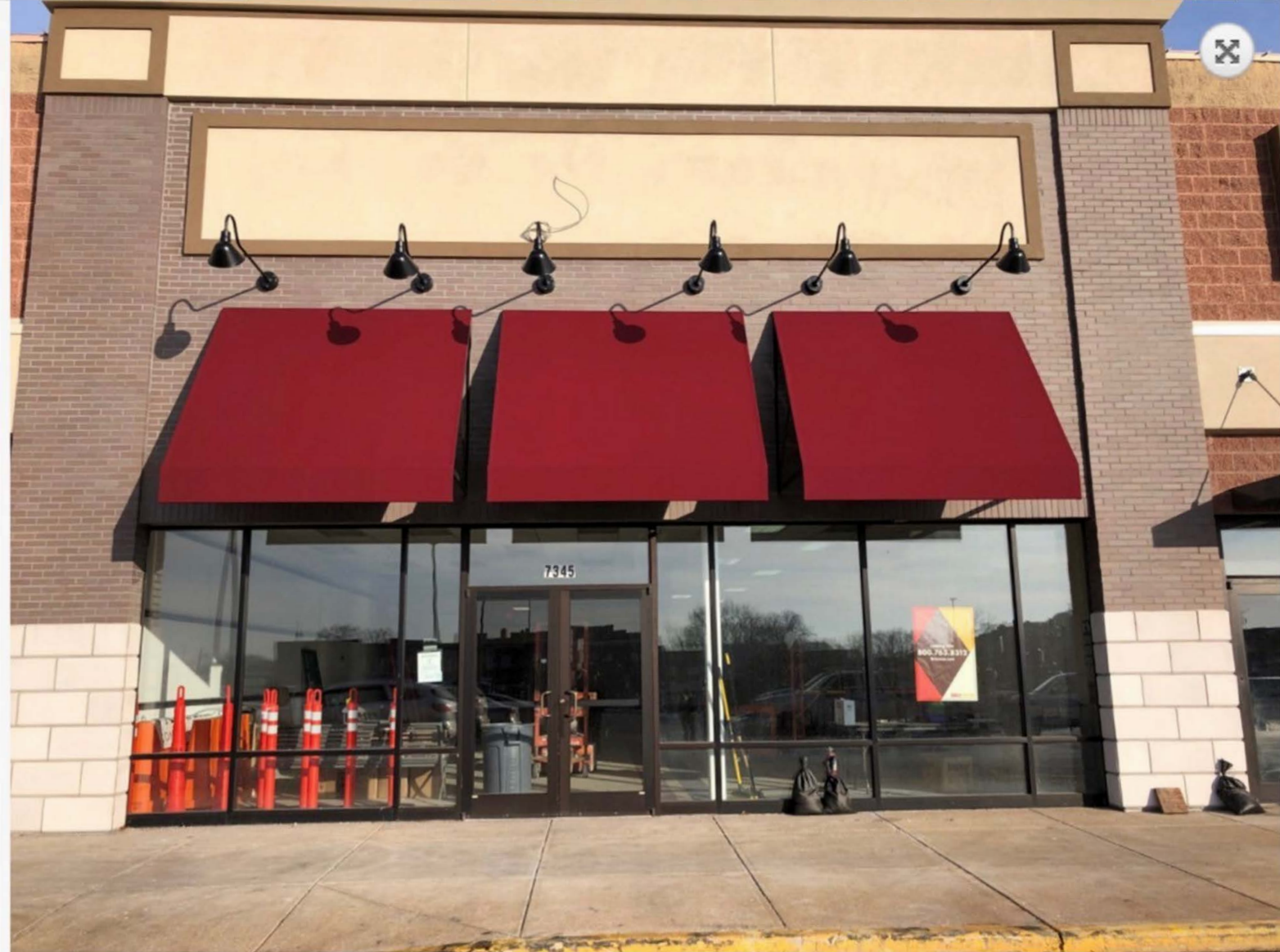
54/127 Slope Mall Storefront Awnings
